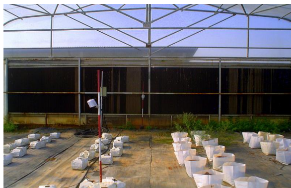
Fig.1: Evaporative pad constructed at the south wall of the greenhouse
